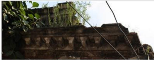
Dentil at roof level (House no: 26)
