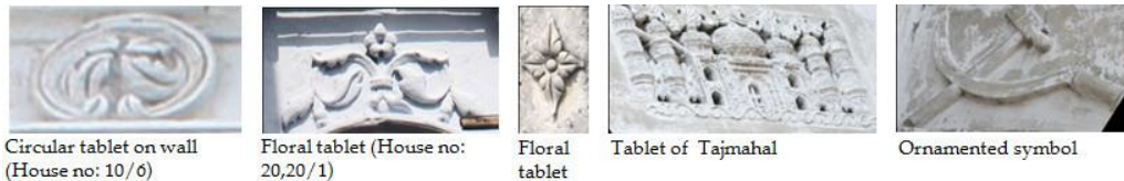
Figure 21: Use of Tablets at Elevation
